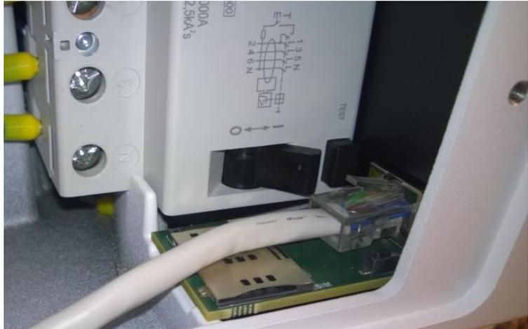
Figure 59: Ethernet UTP cable connected to the connector next to the protection element (RCD in this case)
