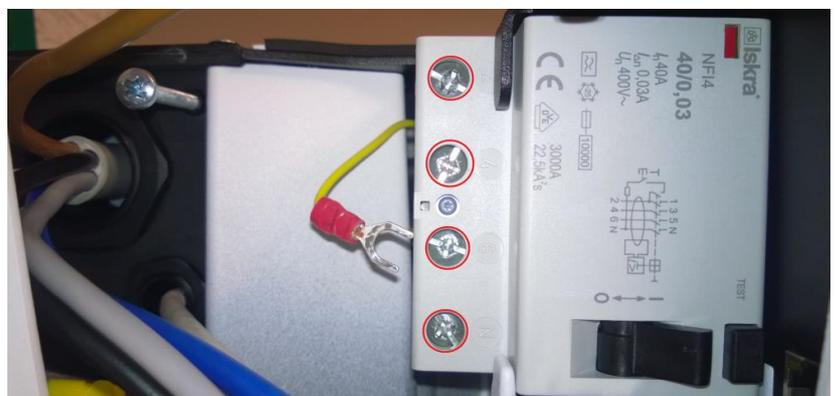
Figure 56: Check that the marked screws are unscrewed so that you can insert the conductors
