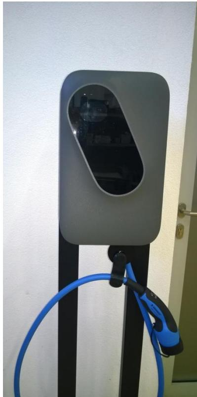
Figure 73: Charging station with short cable
