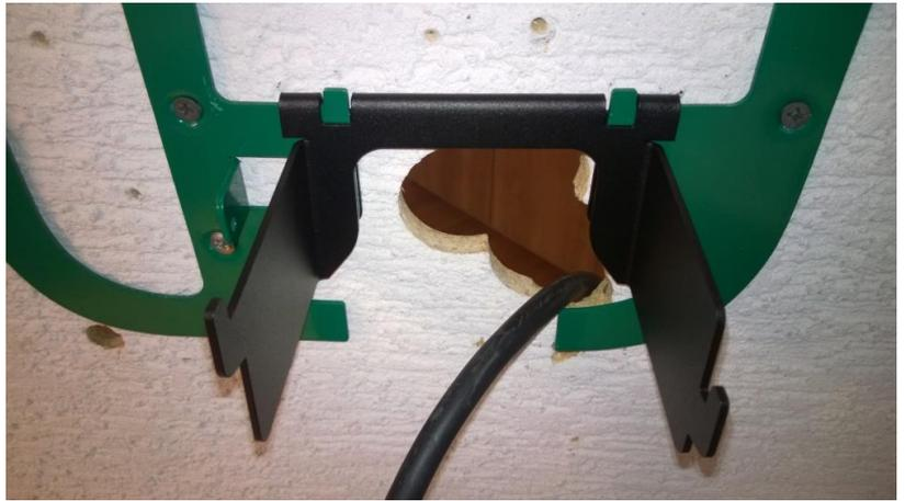
Figure 27: Bracket fasten on to the wall with the installation holder in its place
